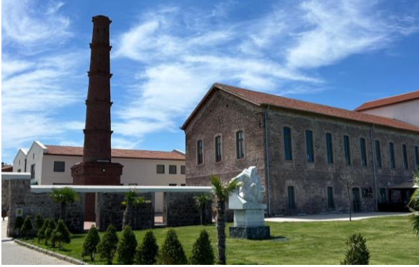
Figure 4. Kırlangıç Olive Oil Factory
